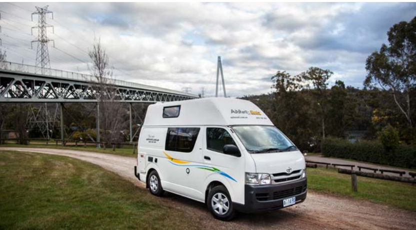
Batman Bridge, Tamar Valley
